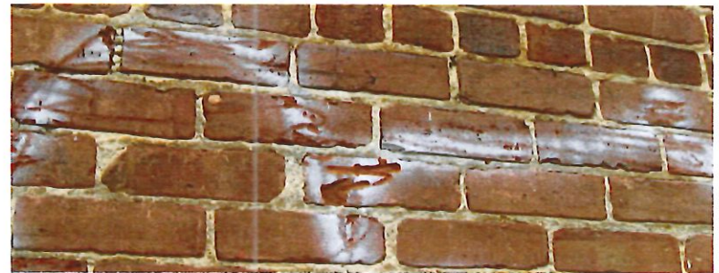
Example of irreversible damage to brick caused by high-pressure washing in an unsuccessful attempt to remove graffiti. (Photo from Easements Atlanta.)
